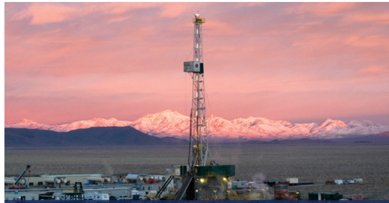
Drilling and power-plant construction at the Blue Mountain geothermal field in Nevada. Photo credit: John Casteel
