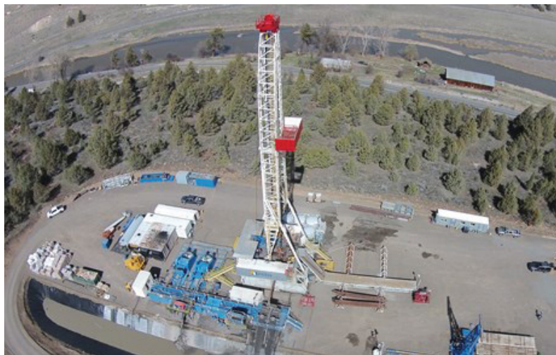
Aerial drone view of geothermal drilling operations near Klamath Falls, Oregon. Photo credit: Kevin P. Graham
