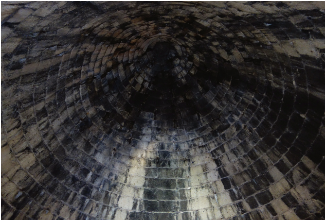
Corbelled vault, Treasury of Atreus, c. 1300-1250 B.C.E., Mycenae, Greece (photo: Steven Zucker, CC BY-NC-SA 2.0)
