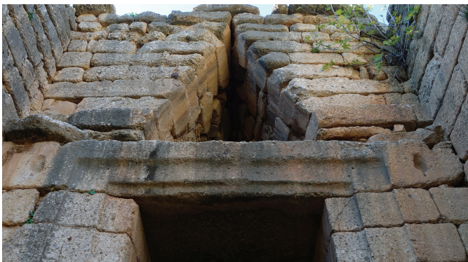
Exterior relieving triangle and lintel, Treasury of Atreus, c. 1300-1250 B.C.E., Mycenae, Greece (photo: Steven Zucker, CC BY-NC-SA 2.0)
