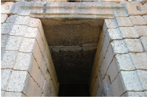
Exterior lintel, Treasury of Atreus, c. 1300-1250 B.C.E., Mycenae, Greece (photo: Steven Zucker, CC BY-NC-SA 2.0)
